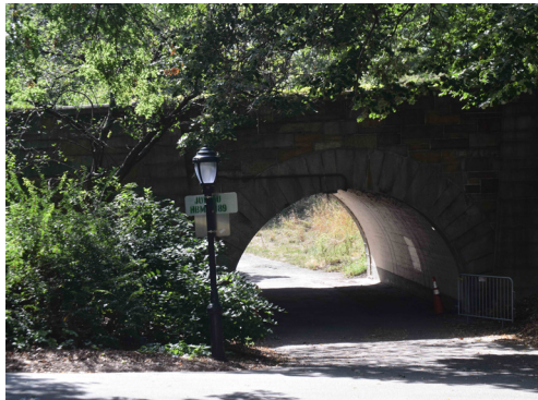
The 79th Street rotunda overhaul is underway.
