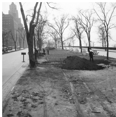
Constructing Riverside Dr.
