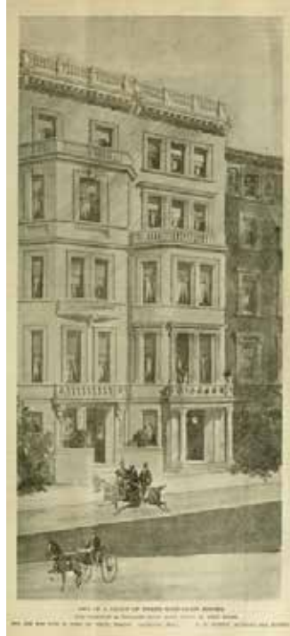
Kight's 5-story row houses
